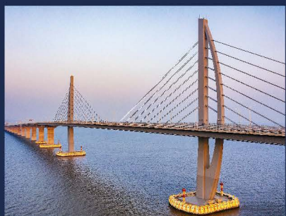
Hong Kong-Zhuhai-Macao Bridge at Macao Port ( Zone B ) 港珠澳大橋澳門口岸(區域B)
